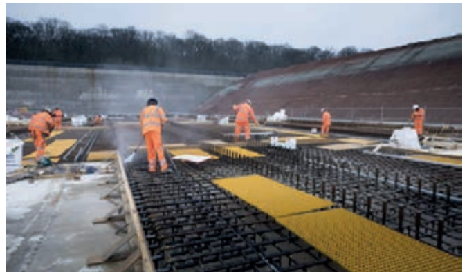
Griptec couplers being used at HS2 Long Itchington Wood Tunnel
