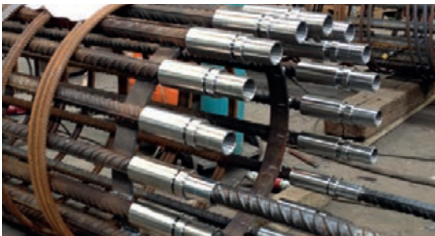
Pile cages using nVent LENTON Position couplers
